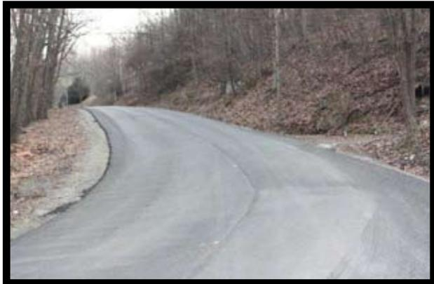
A J.F. Allen Co. vibratory padfoot roller immediately compacted the mixture to the project density requirements and its motor grader then shaped the areas to project grades and cross slope for final grade. Final compaction was then accomplished with a double-drum steel-wheel roller to seal up the newly-reclaimed material and to maximize smoothness.
