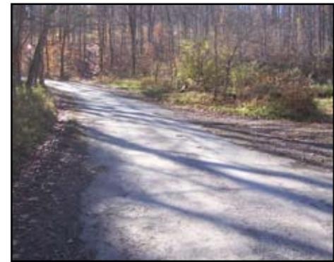
Photos from SR 80 (Prickett’s Creek Rd.) shows the full extent of the damage caused by a combination of poor subgrade, heavy loads and the age of the road.
