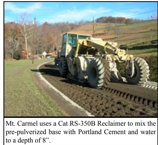
Mt. Carmel uses a Cat RS-350B Reclaimer to mix the pre-pulverized base with Portland Cement and water to a depth of 8".
