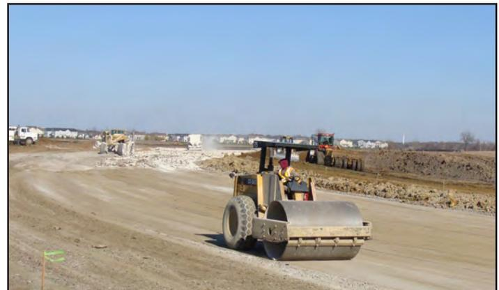
The last step in the soil stabilization process is final compaction and sealing with a smooth drum roller.
