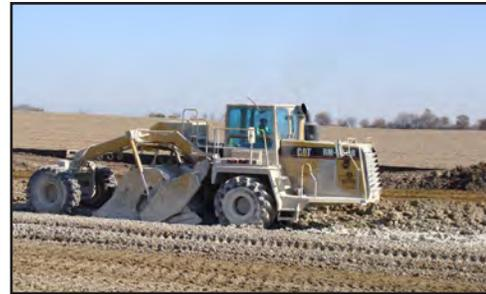
The Caterpillar RM 350 Road Reclaimer mixes lime and soil 16” deep. Mt. Carmel maintains a fleet of 28 various makes and models of similar machines for soil stabilization.
