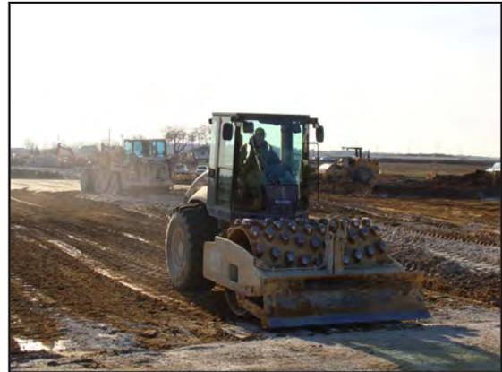
Mt. Carmel uses a Cat vibratory pad foot roller for initial compaction of the lime modified soil.
