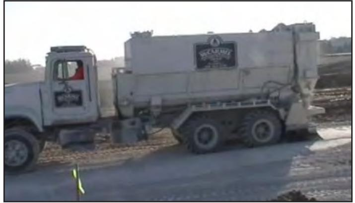
Lime Kiln Dust is an extremely fine, lightweight, dry powder. On this job, a 5% application rate was used. This amounts to 65 lbs. of LKD spread per square yard. This spread rate is controlled by the truck operator and accuracy is critical for a high quality end product.
