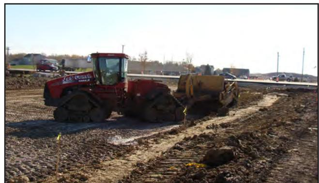
Just a short time after Mt. Carmel finished treating this area, J&S is already placing the next lift on the south end of Municipal Dr. This same area was rutting under light loads just hours before.
