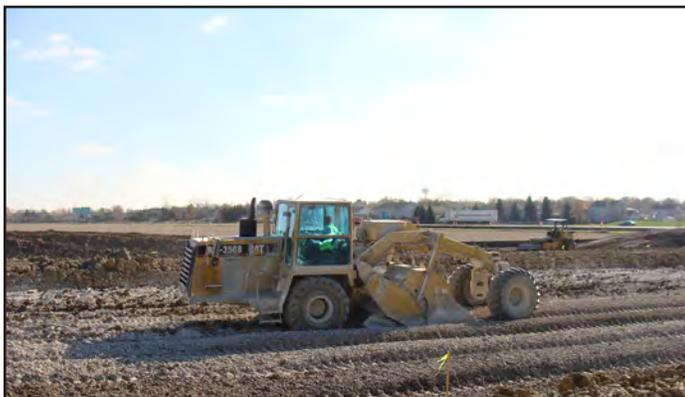
The Cat RM 350 and other similar machines designed for stabilization applications is the only way to thoroughly blend and pulverize the lime and soil. Thorough mixing is critical to the performance of the treated soil. Discs should never be used for soil stabilization.
