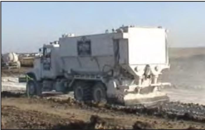
All of Mt. Carmel's 65 spreader trucks are designed and custom built in house by their people. The trucks that Mt. Carmel used on this job are equipped with a patented dust collection system that captures fugitive dust and sends it back to the material hopper.
