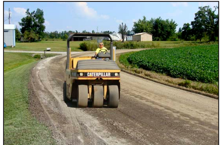
Following remixing, the area is compacted with a sheepsfoot roller and shaped to grade before a pneumatic roller finishes the job. The new cement stabilized base is ready for the surface.
