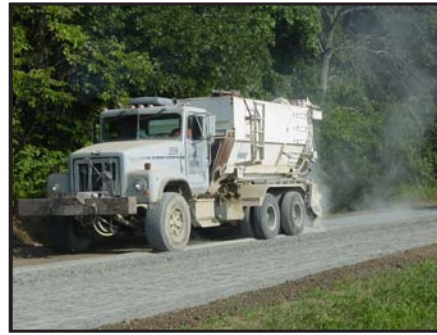
Portland Cement is then applied at the specified application rate using Mt. Carmel's custom built spreader trucks which are specially designed for accuracy and dust control. For this project, Mt. Carmel used 6% cement.
