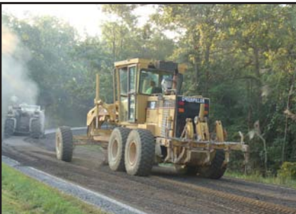
The first step in FDR is to pulverize the existing roadway. The resulting gradation is 90% < 1".
