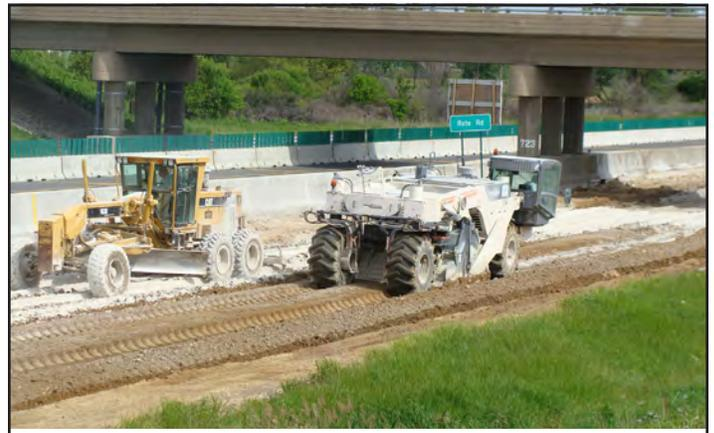
Mt. Carmel uses a Wirtgen 2400 Reclaimer to mix the lime and subgrade soil thoroughly to a depth of 16" before compaction. This mixing equipment is built for soil stabilization applications and is critical to the performance of the operation and the end product.
