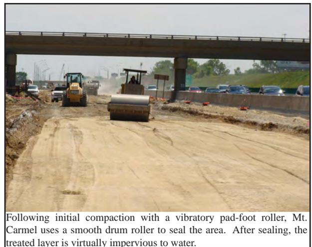
Following initial compaction with a vibratory pad-foot roller, Mt. Carmel uses a smooth drum roller to seal the area. After sealing, the treated layer is virtually impervious to water.
