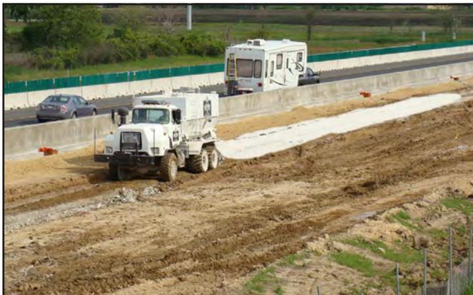
For this project, Mt. Carmel utilized 2 spreaders from their fleet of 65 that contain a patented dust collection system designed to minimize fugitive dust during spreading. Mt. Carmel builds all of their spreading equipment in house to ensure they are built to the highest standards.
