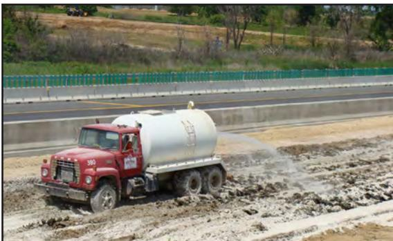
Believe it or not... Mt. Carmel actually has to add water to the lime kiln dust due to the tremendous drying effects of lime products.
